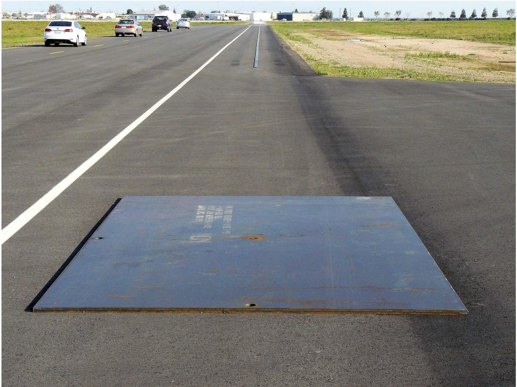
Figure A9. Steel Trench Plate
