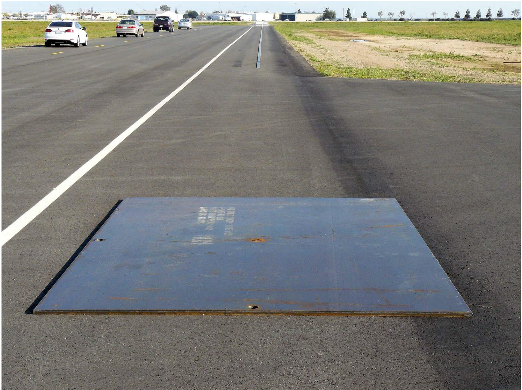
Figure A9. Steel Trench Plate
