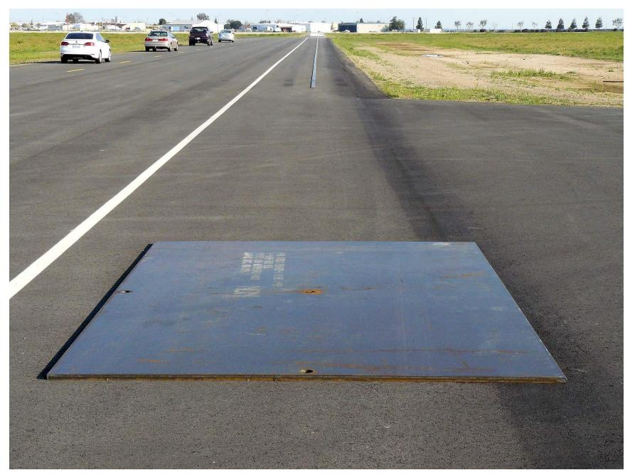
Figure A9. Steel Trench Plate
