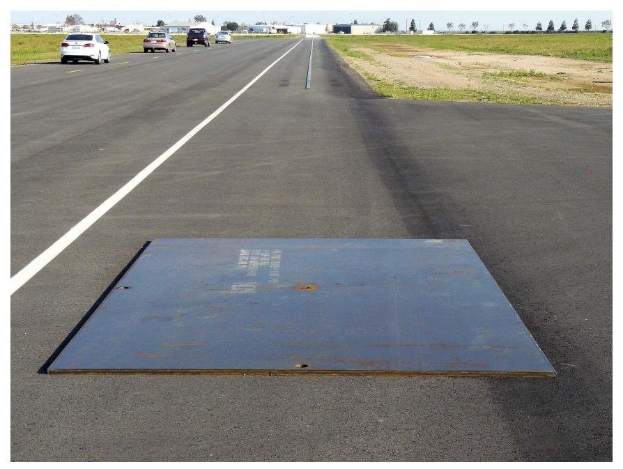
Figure A9. Steel Trench Plate A-11
