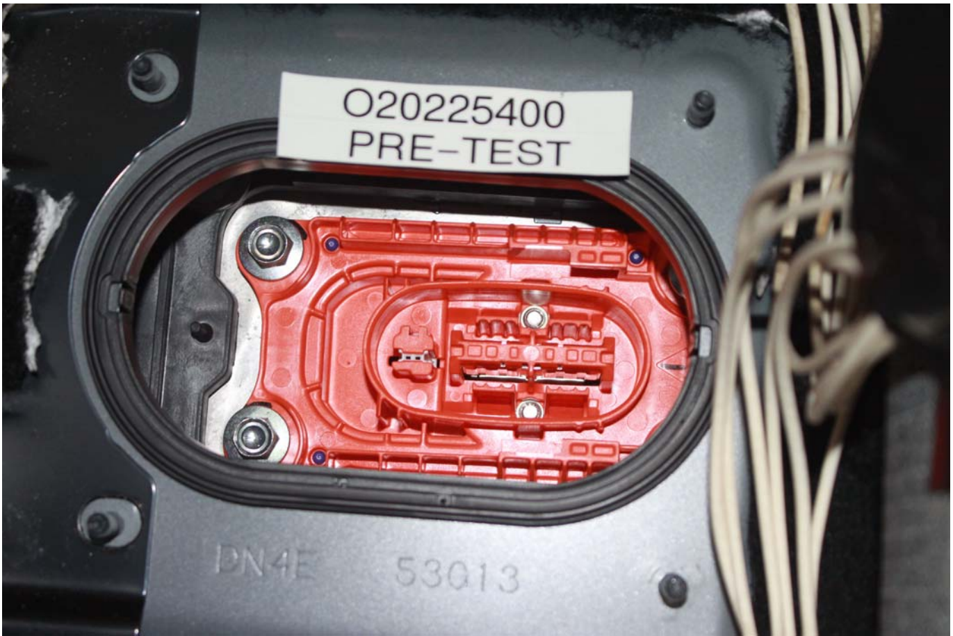
Photo No. 305-08 - Manual High Voltage Service Disconnect Removed
