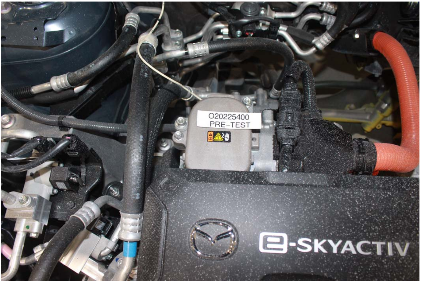
Photo No. 305-02 - Power Inverter Warning Label
