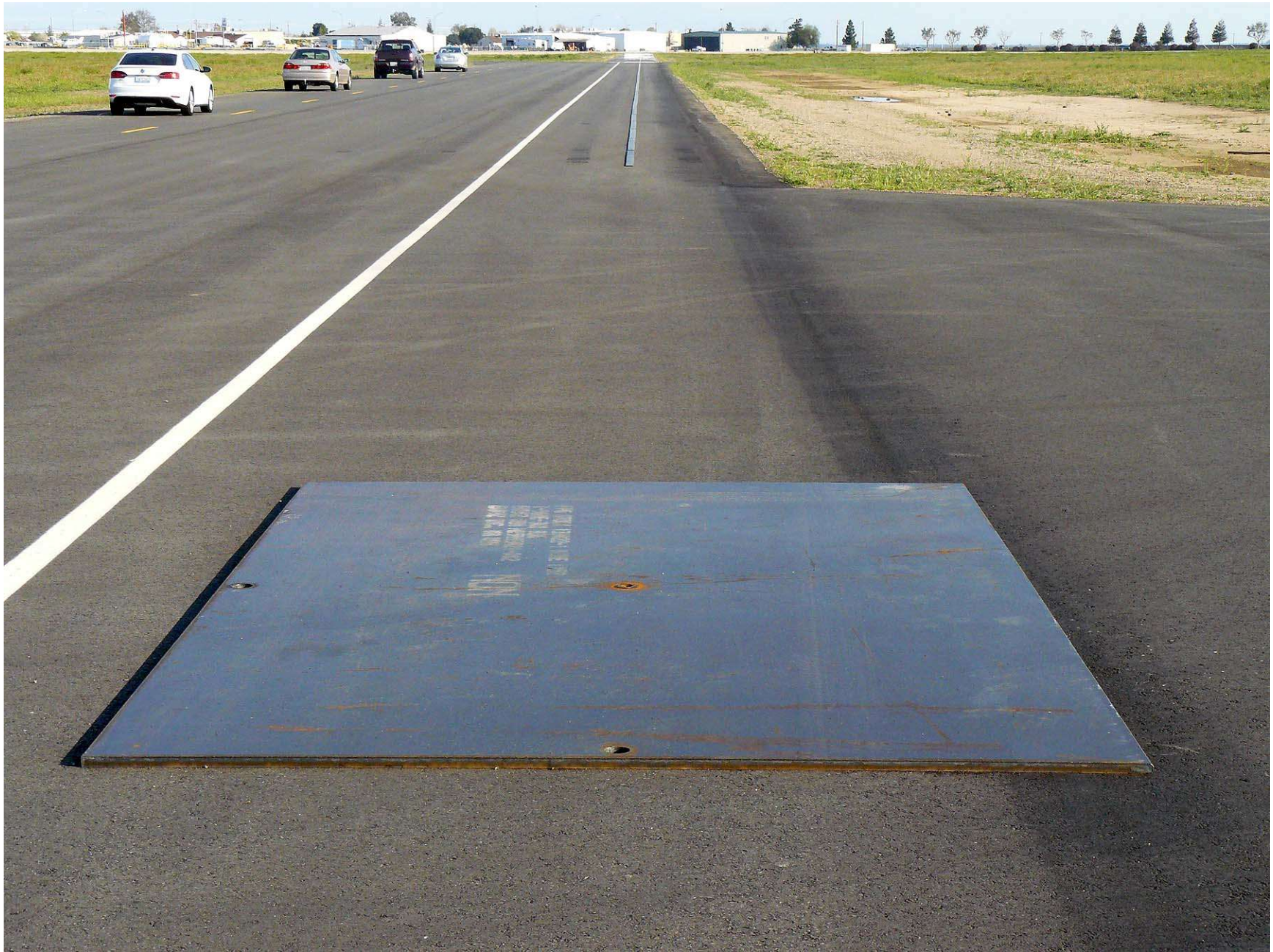
Figure A9. Steel Trench Plate
