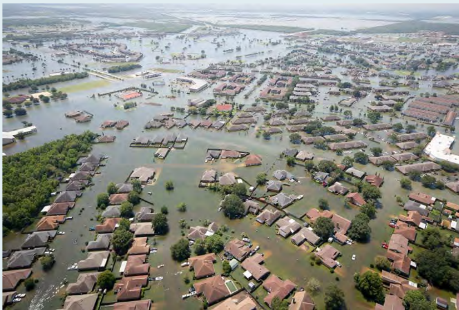
Figure 17.2: Hurricane Harvey led to widespread flooding and knocked out power to 300,000 customers in Texas in 2017, with cascading effects on critical infrastructure facilities such as hospitals, water and wastewater treatment plants, and refineries. The photo shows Port Arthur, Texas, on August 31, 2017—six days after Hurricane Harvey made landfall along the Gulf Coast. Photo credit: Staff Sgt. Daniel J. Martinez, U.S. Air National Guard.
