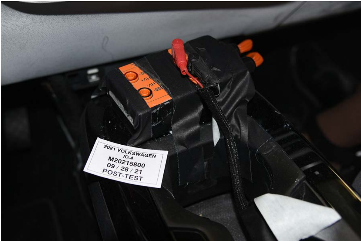
FIGURE 305-027. Post-Impact View of Other Test Devices
