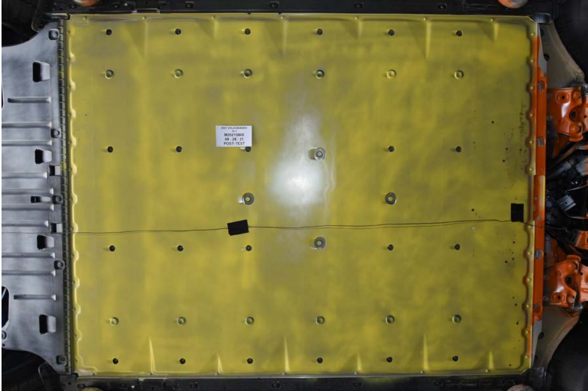
FIGURE 305-013. Post-Impact View of Battery Box(s) or Container(s) Which Holds Individual Battery Modules
