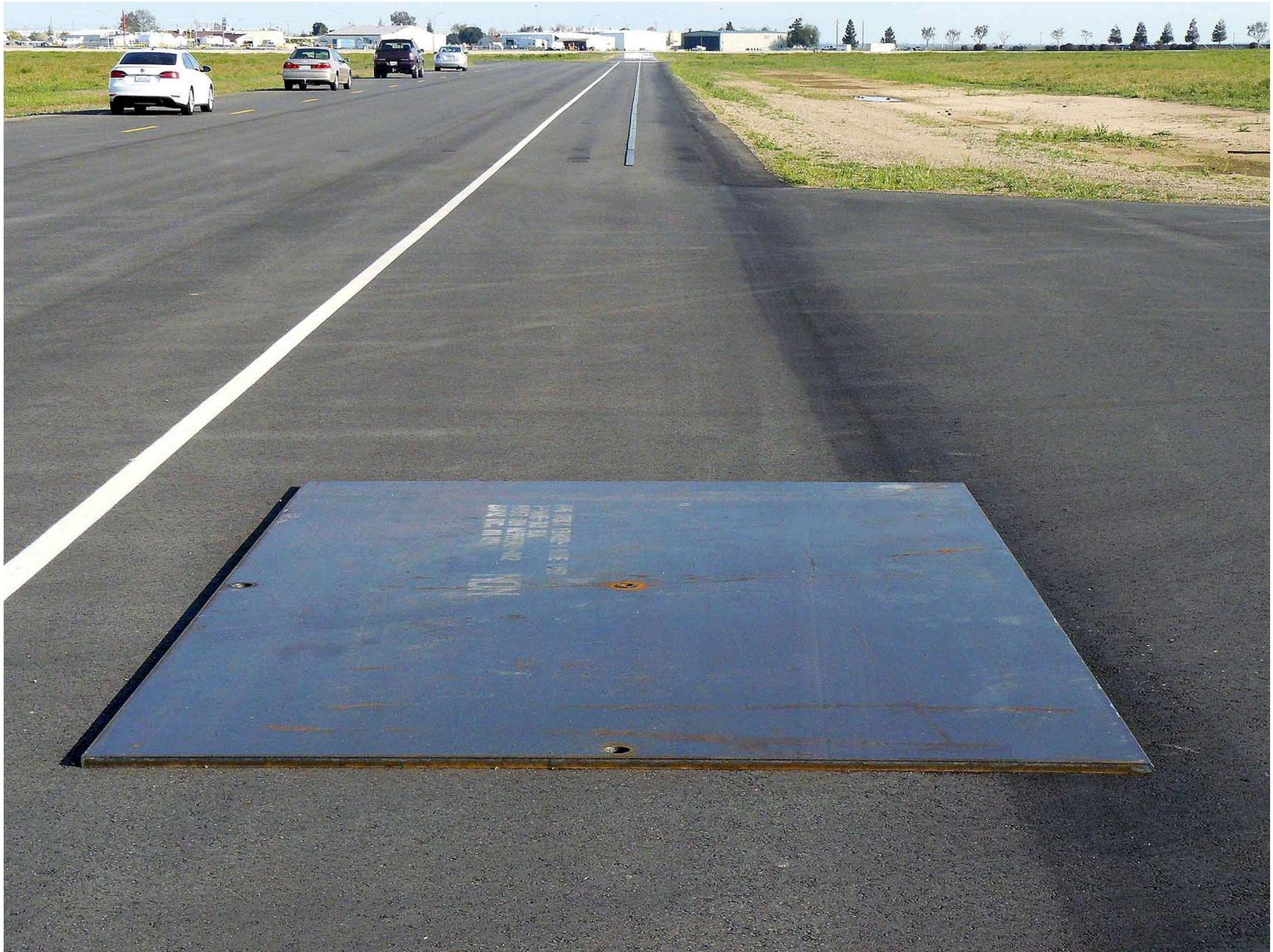
Figure A9. Steel Trench Plate
