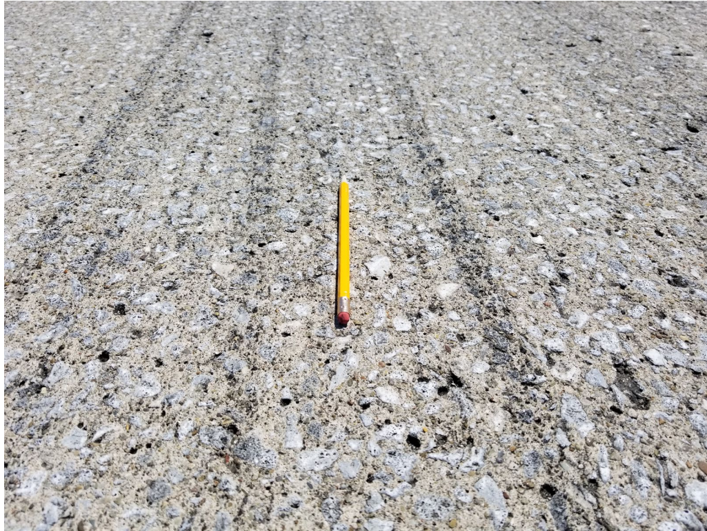
Broomed Concrete Close-up
