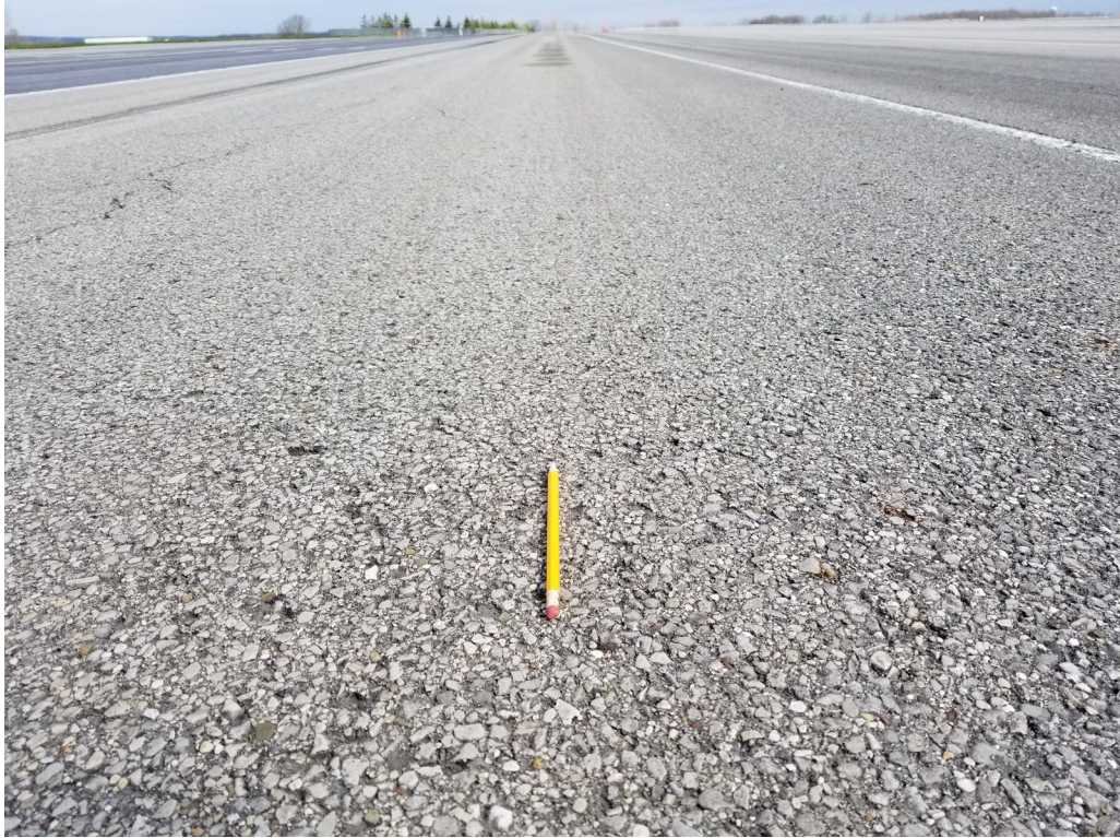
Wet Asphalt Pad
