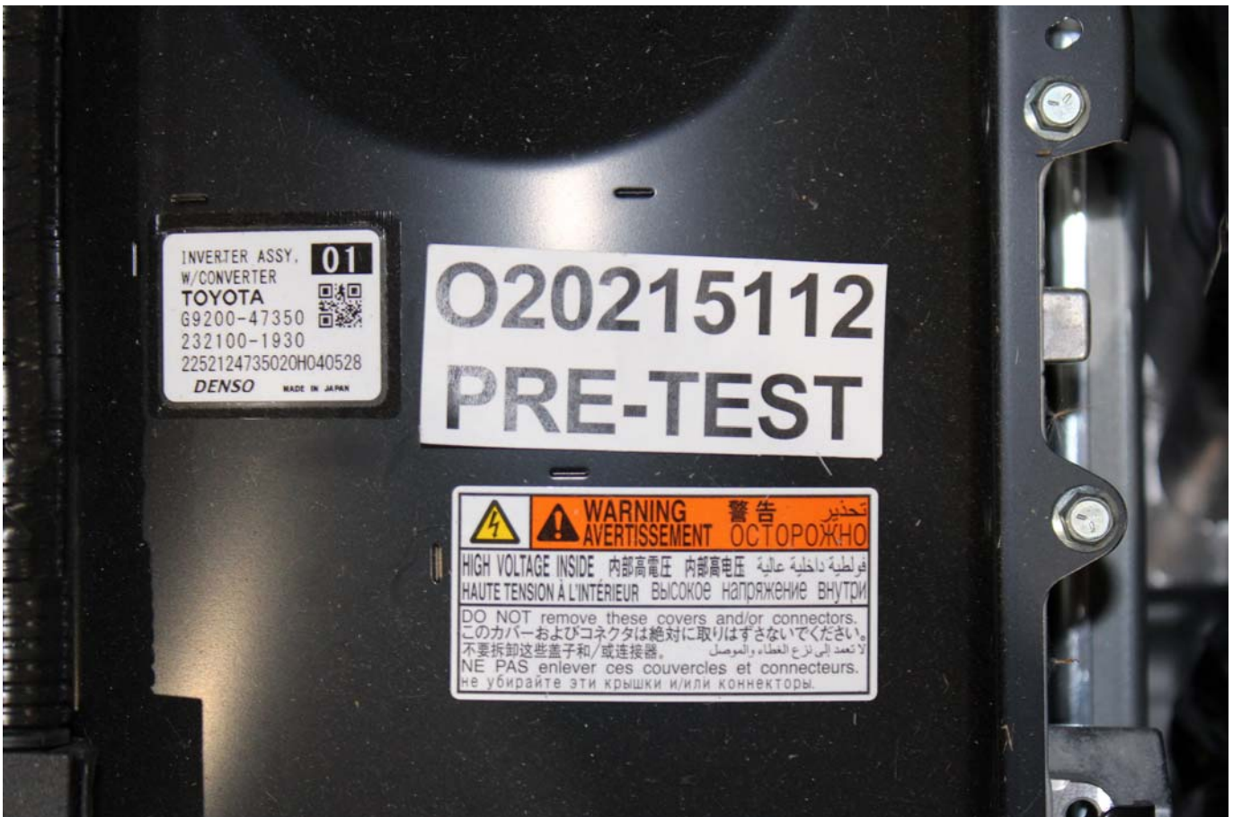
Photo No. 305-02 - Power Inverter Warning Label
