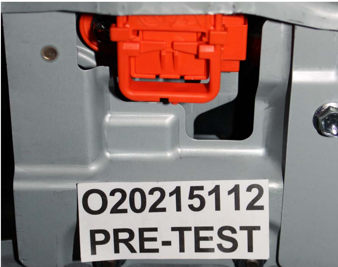
Photo No. 305-06 - Manual High Voltage Service Disconnect in Place
