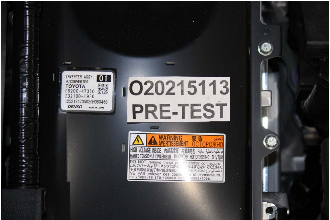
Photo No. 305-02 - Power Inverter Warning Label
