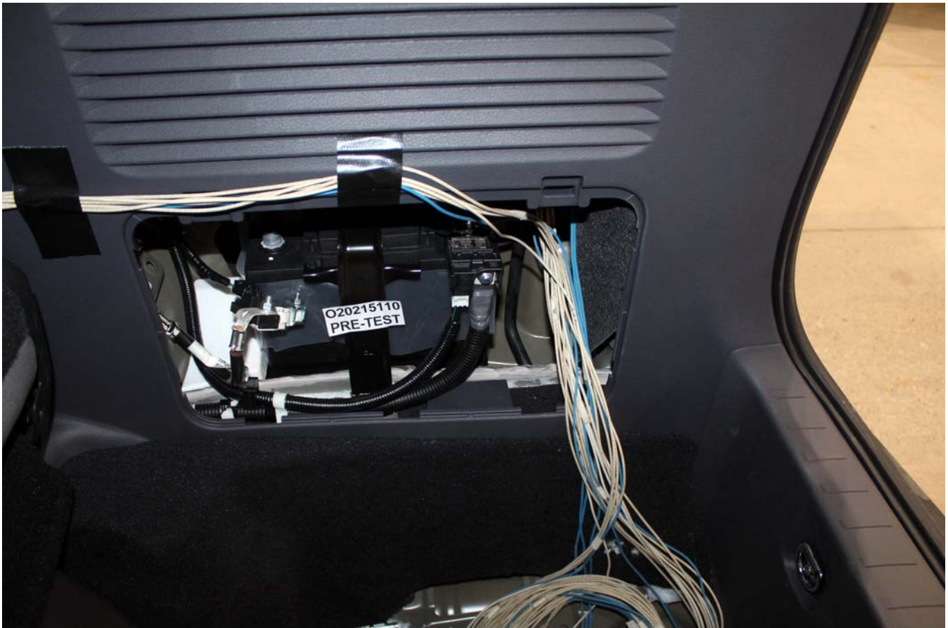
Photo No. 305-01 - Auxiliary Power Module Warning Label
