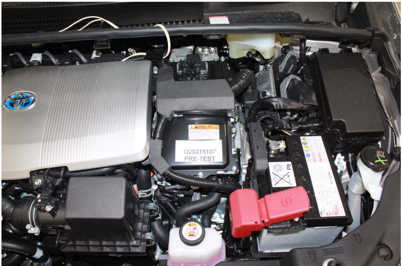
Photo No. 305-01 - Auxiliary Power Module Warning Label
