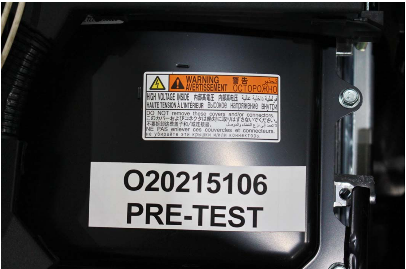
Photo No. 305-02 - Power Inverter Warning Label
