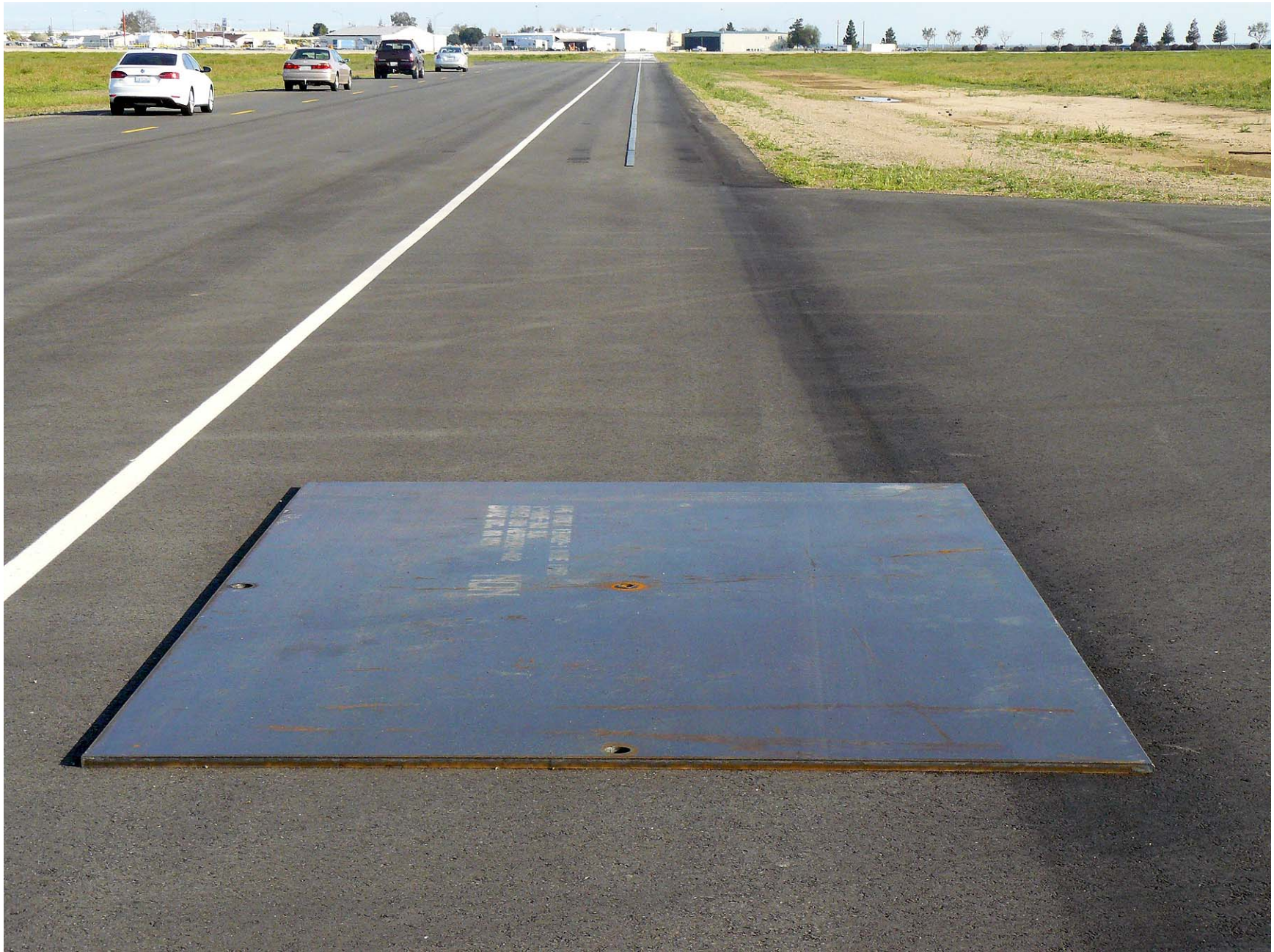
Figure A9. Steel Trench Plate A-11
