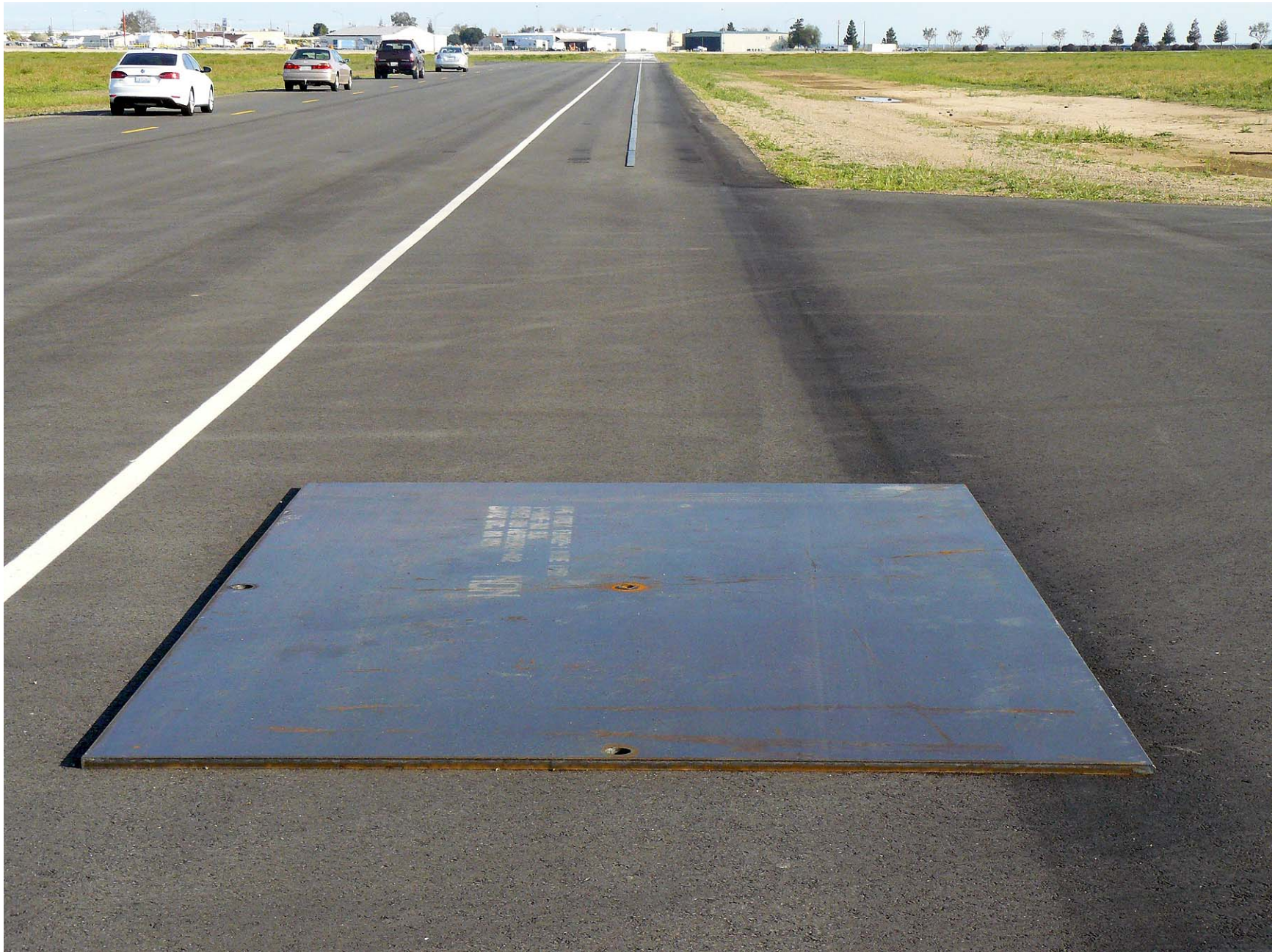
Figure A9. Steel Trench Plate
