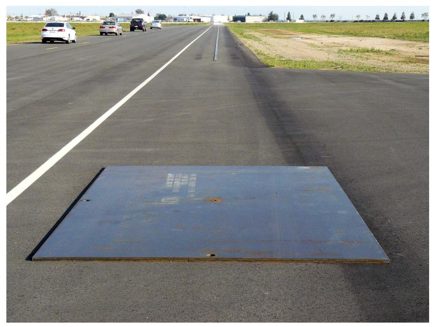
Figure A9. Steel Trench Plate
