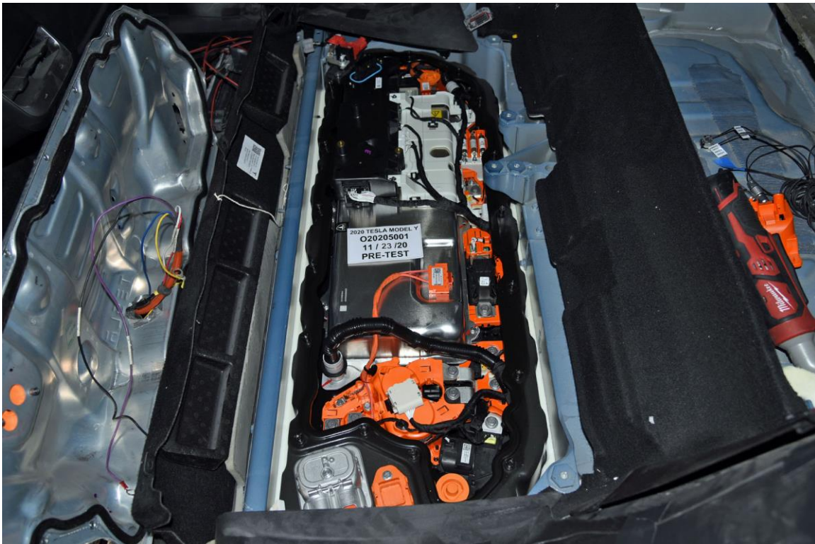
FIGURE 305-020. Pre-Impact View of Other Visible Electric Propulsion Components Note: Date on Placard Should Read 11/23/20
