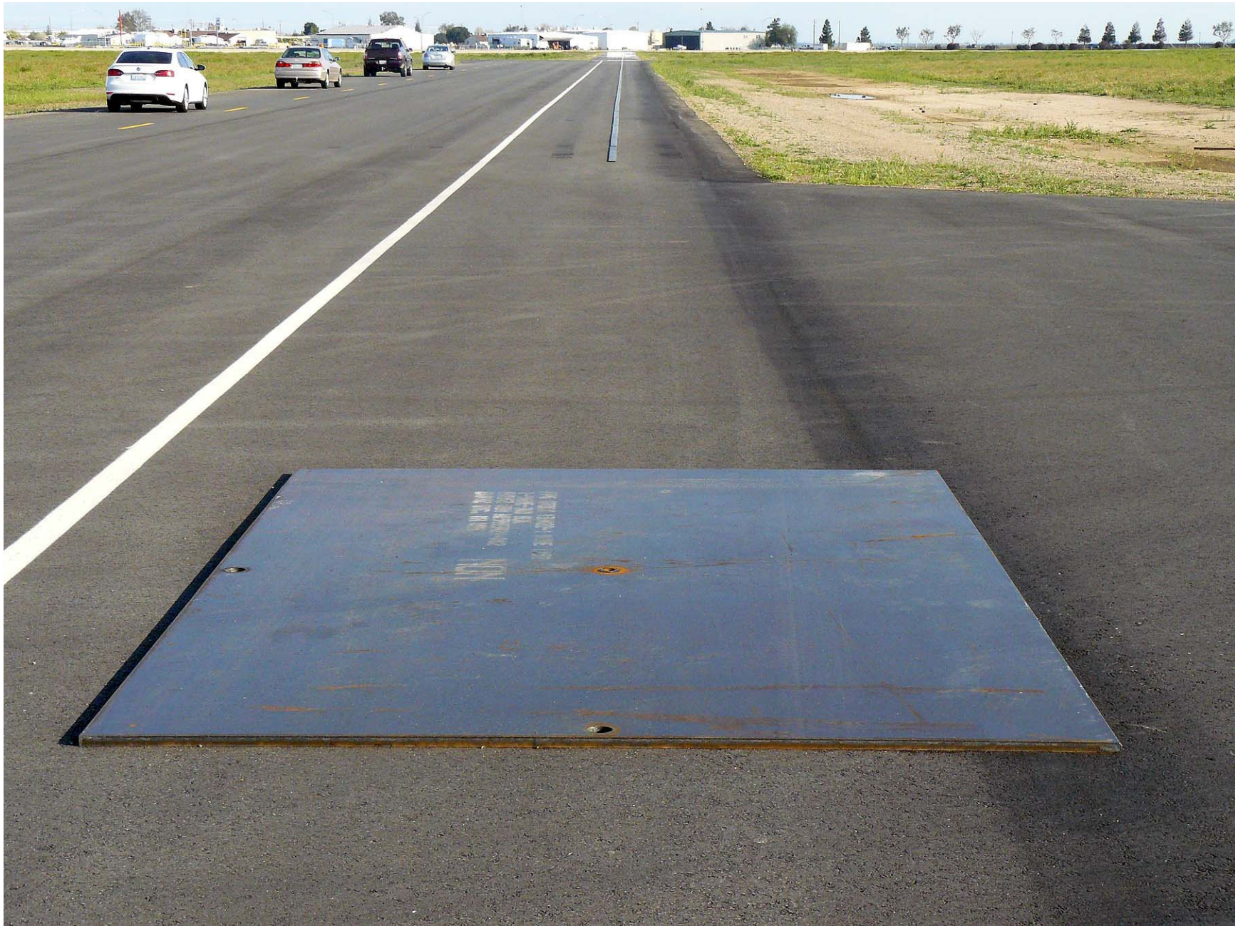
Figure A9. Steel Trench Plate
