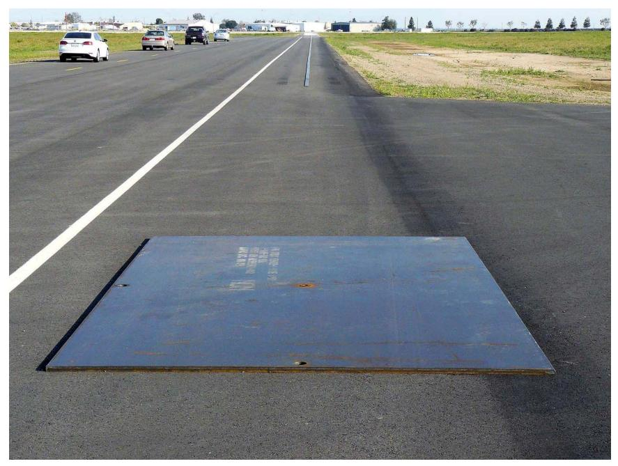
Figure A9. Steel Trench Plate
