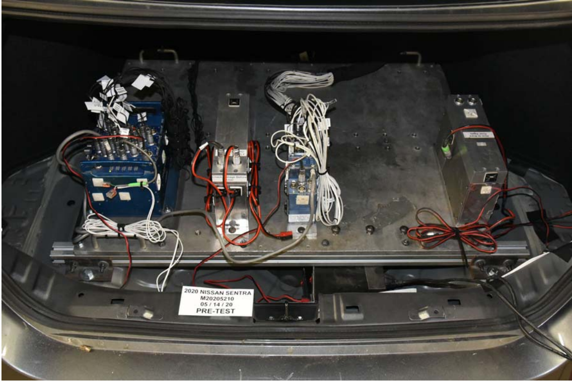
FIGURE 61. Pre-Test Ballast View
