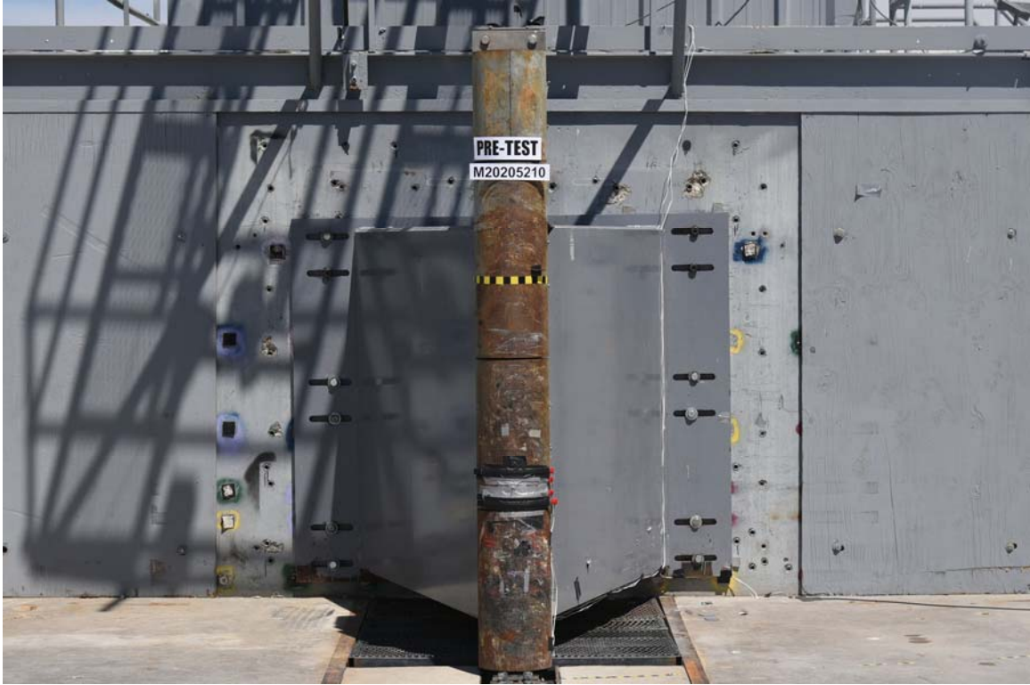
FIGURE 57. Pre-Test Pole Barrier Front View
