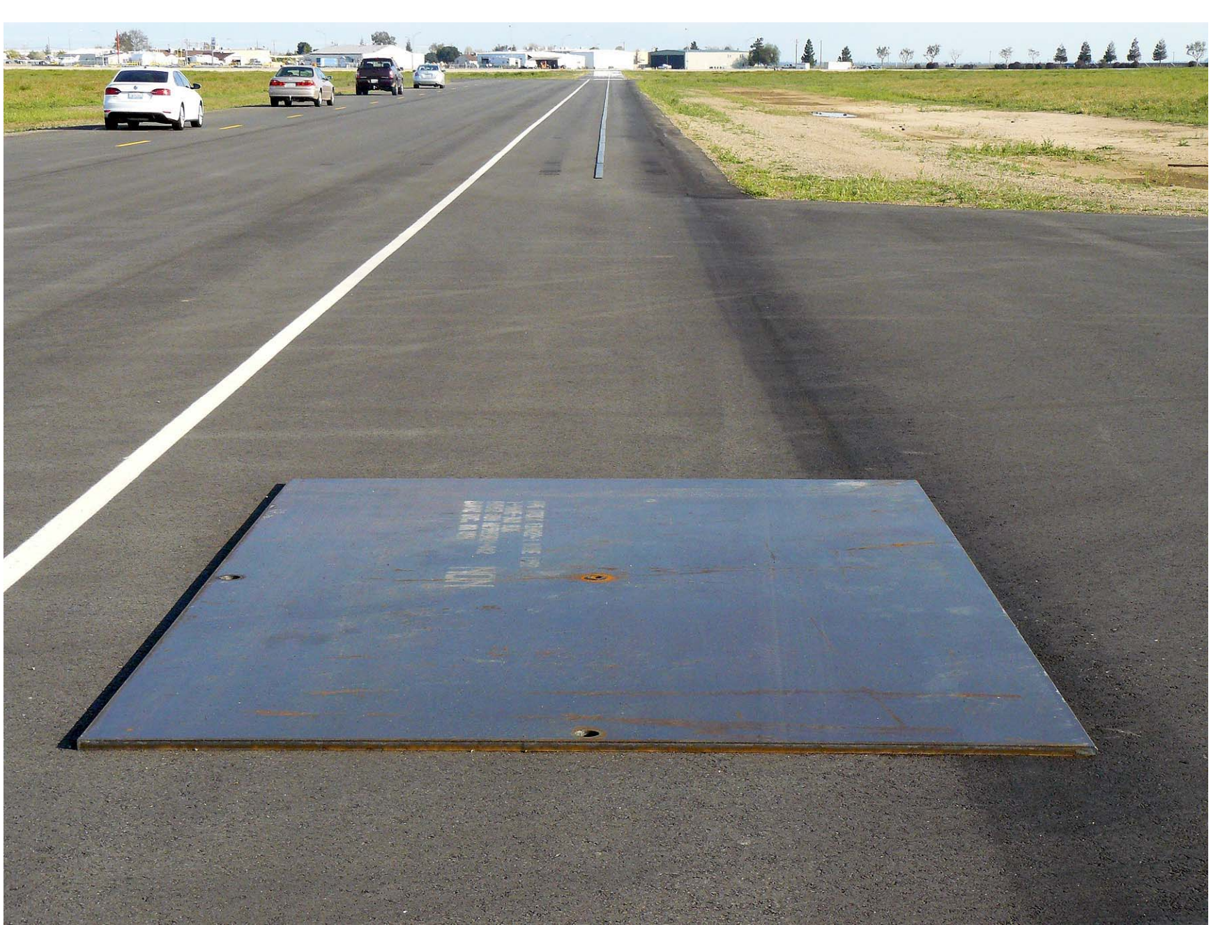
Figure A9. Steel Trench Plate
