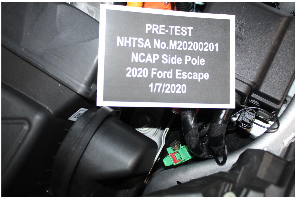
Figure A-6: Manual High Voltage Service Disconnect Removed (Plug)
