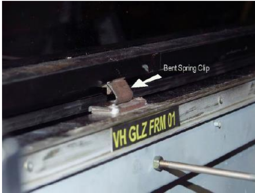
Figure 13 Van Hool primary latch spring clip bending failure (Fig. 5.18 of reference 1)
