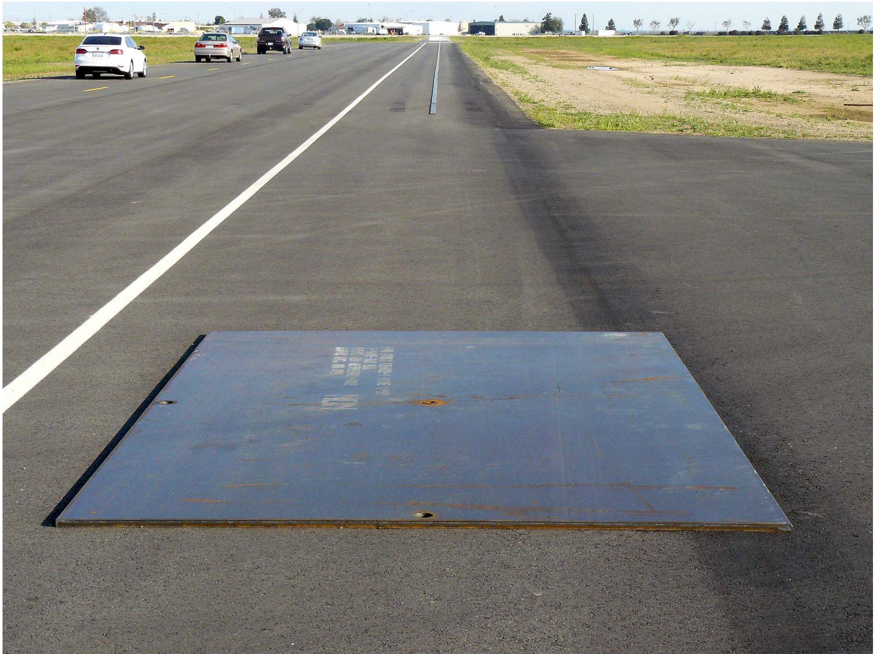
Figure A9. Steel Trench Plate
