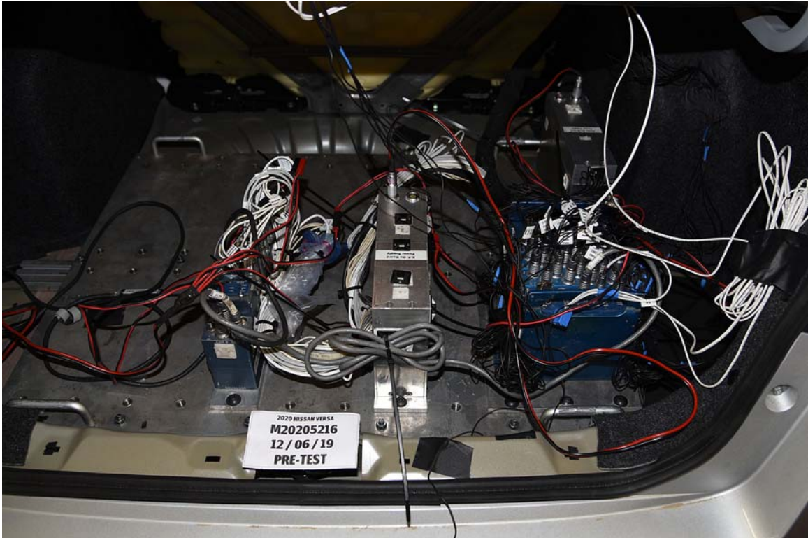
FIGURE 61. Pre-Test Ballast View
