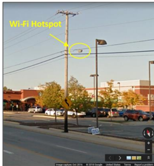
Figure 3: Outdoor Wi-Fi Hotspot Roadside Installation
