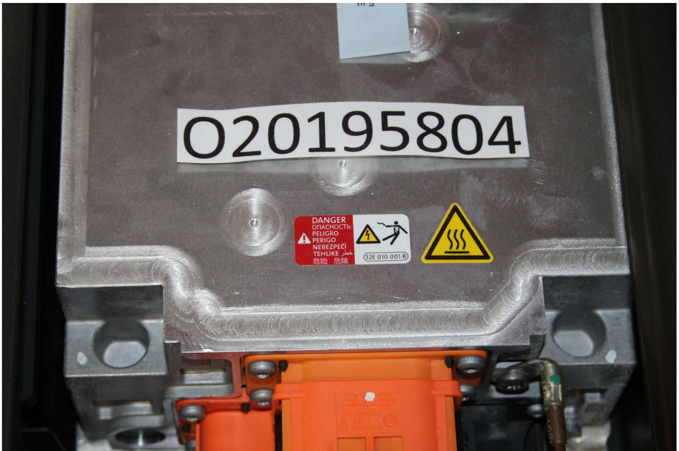
Photo No. 002 - Power Inverter Warning Label
