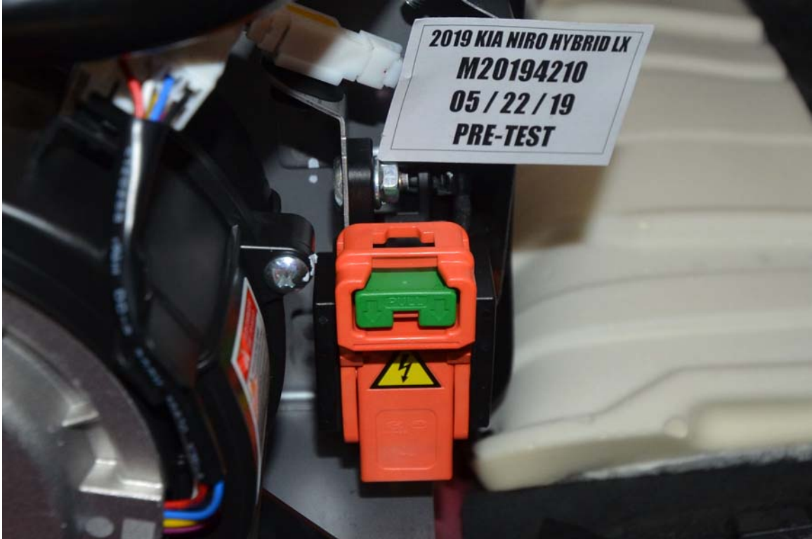
FIGURE 6. Manual High Voltage Service Disconnect in Place
