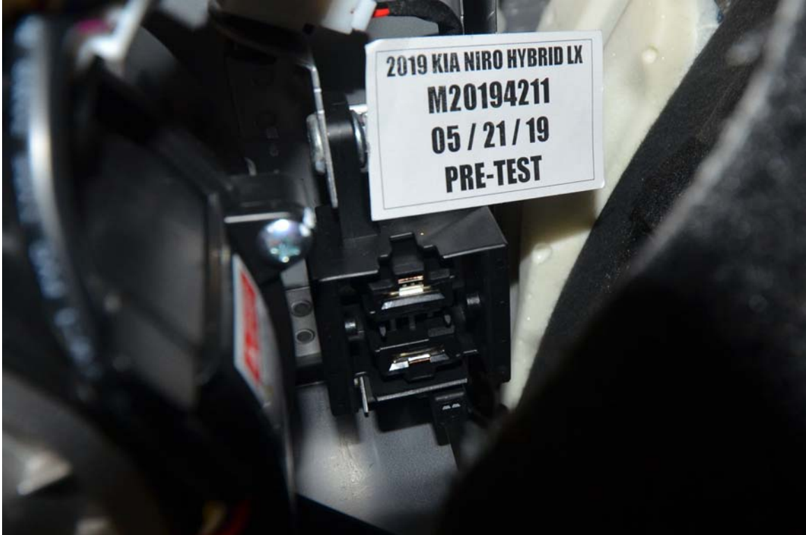
FIGURE 8. Manual High Voltage Service Disconnect Removed
