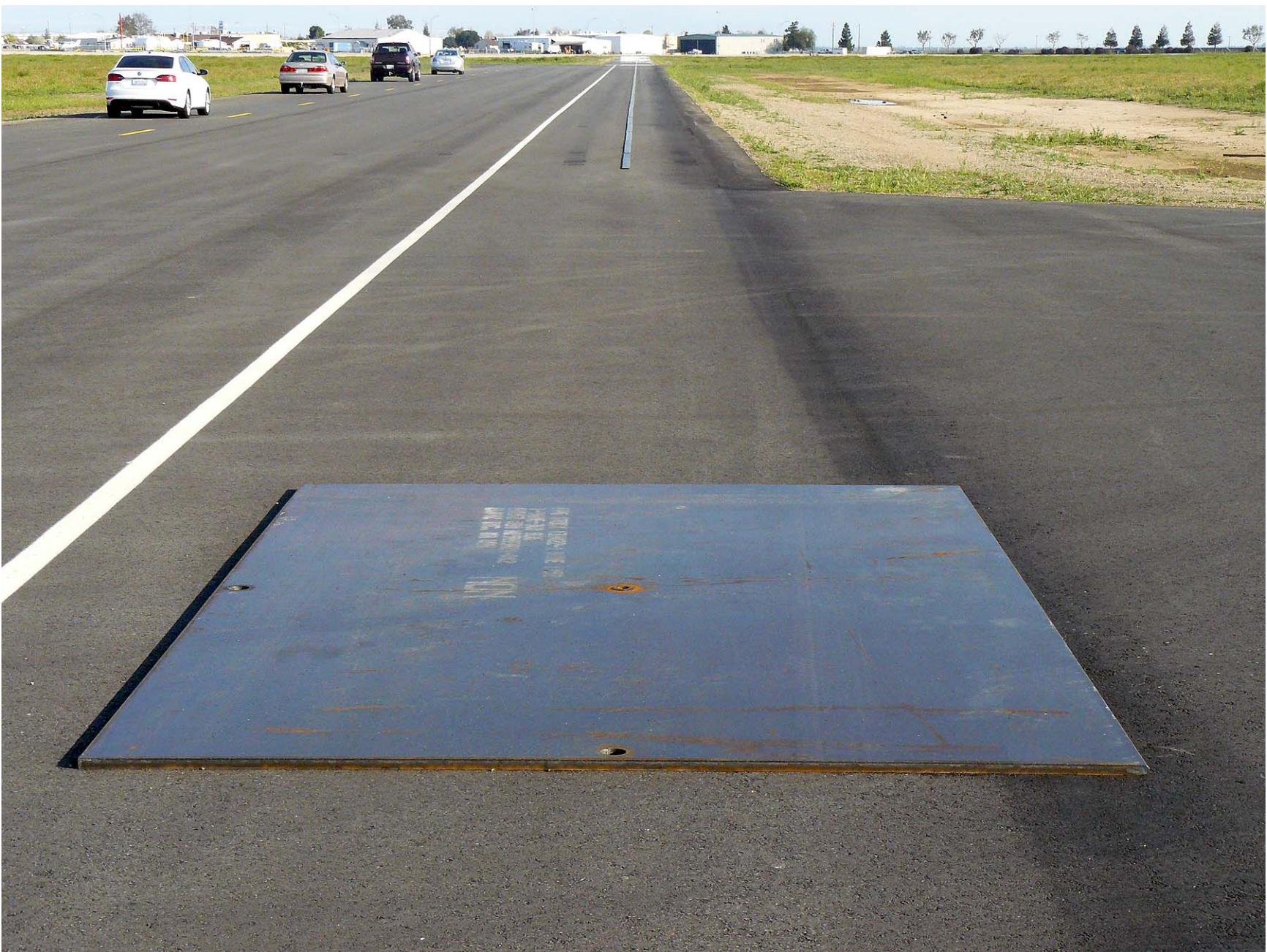
Figure A9. Steel Trench Plate
