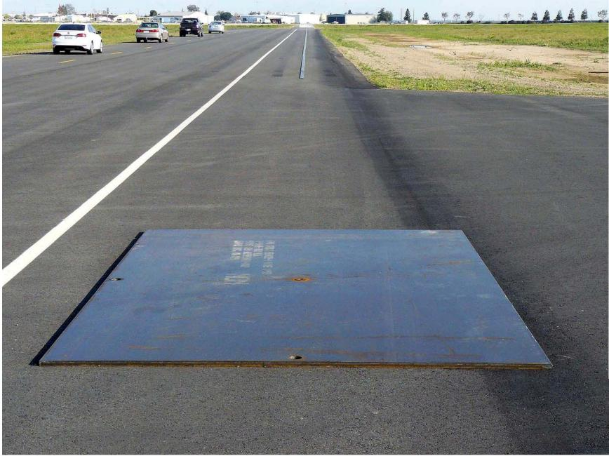
Figure A9. Steel Trench Plate
