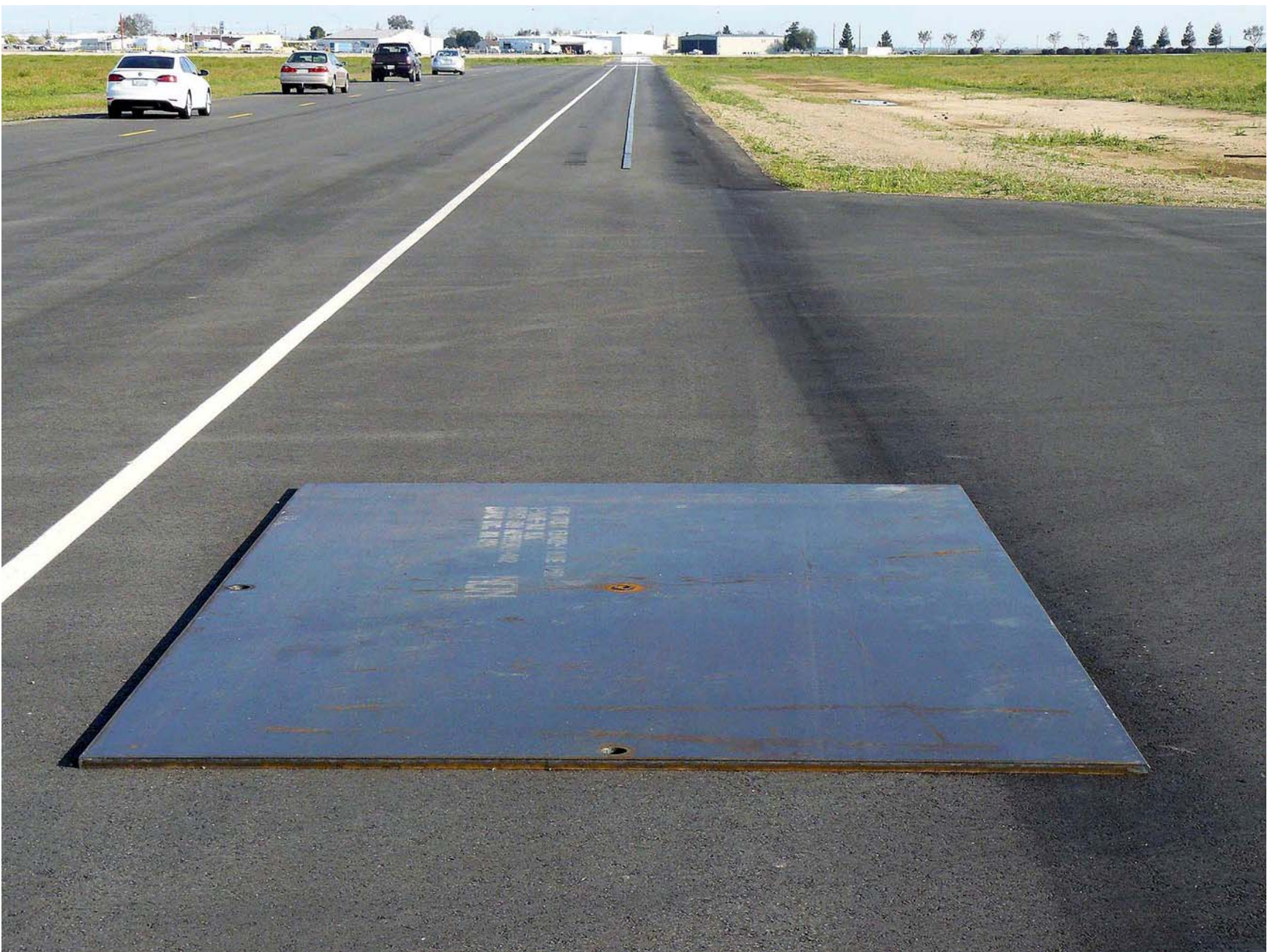
Figure A9. Steel Trench Plate
