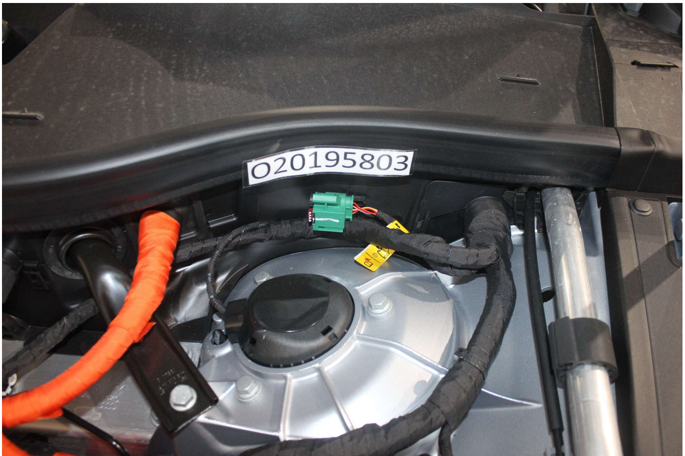
Photo No. 305-006 - Manual High Voltage Service Disconnect in Place
