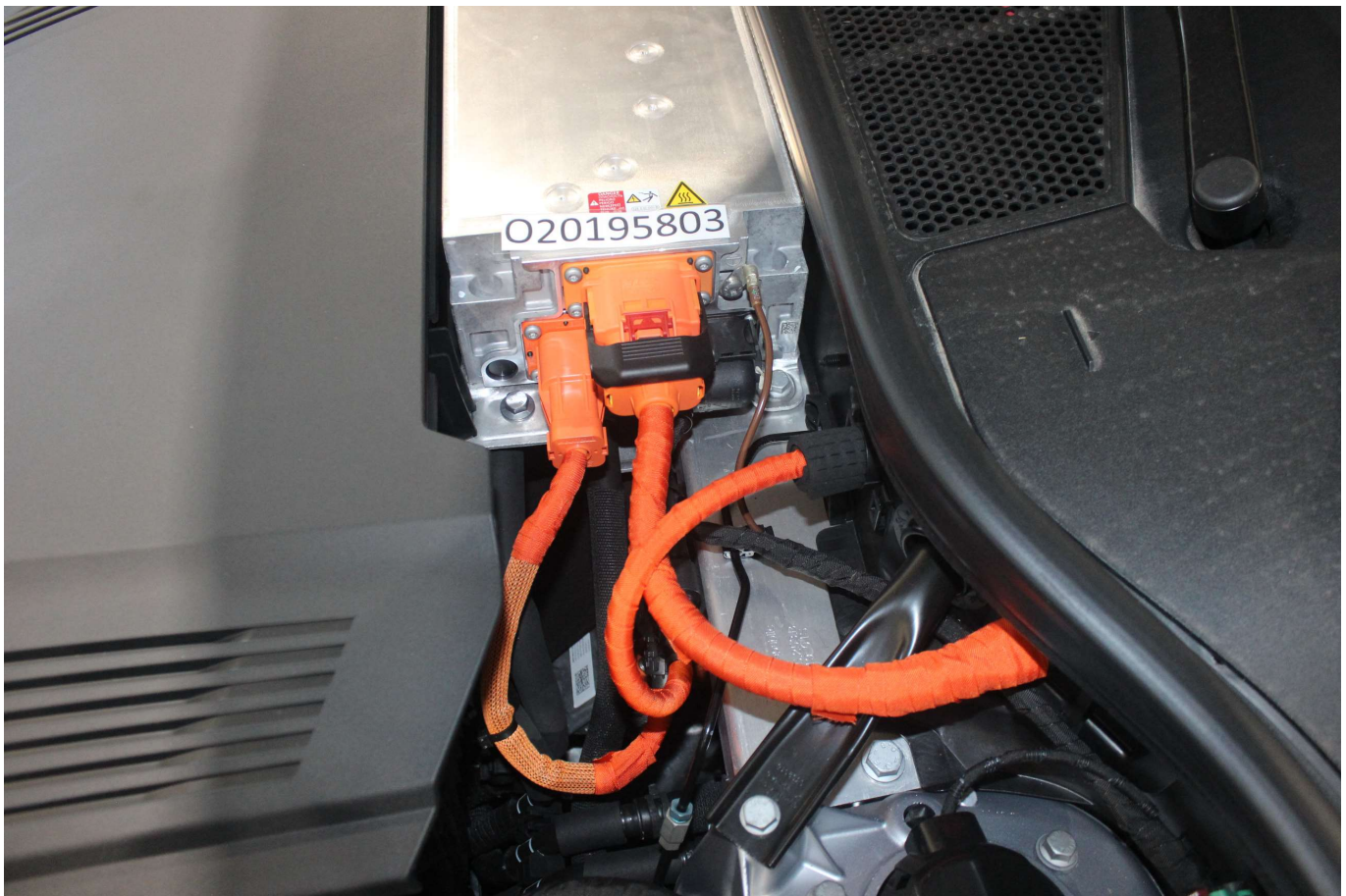
Photo No. 305-018 - Pre-Impact View of High Voltage Interconnect(s)
