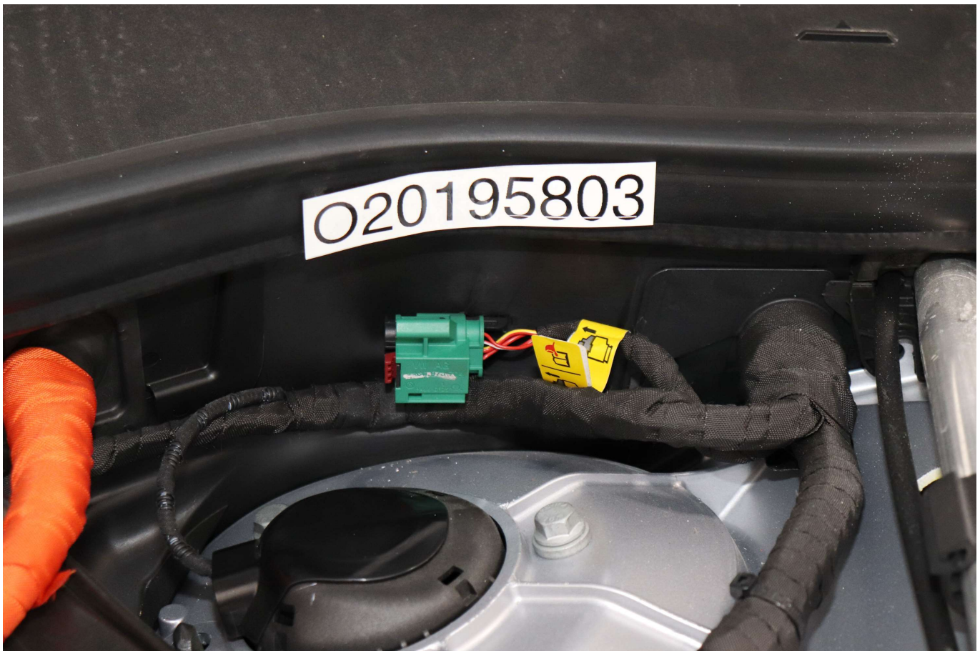
Photo No. 305-003 - First Responder Warning Label
