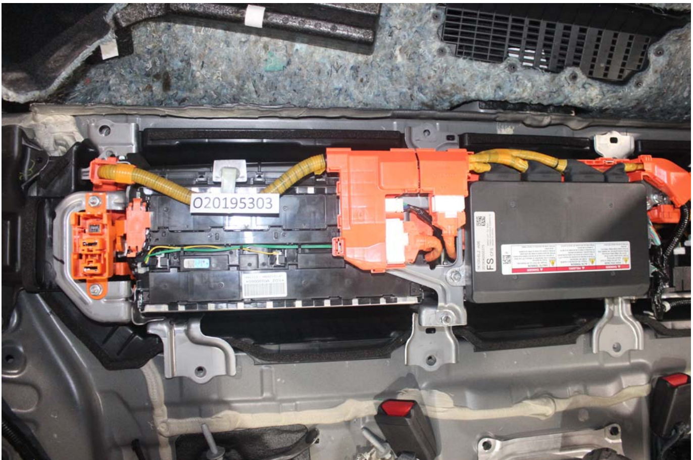
Photo No. 011 - Pre-Impact View of Battery Box(s) or Container(s) Which Holds Individual Battery Modules
