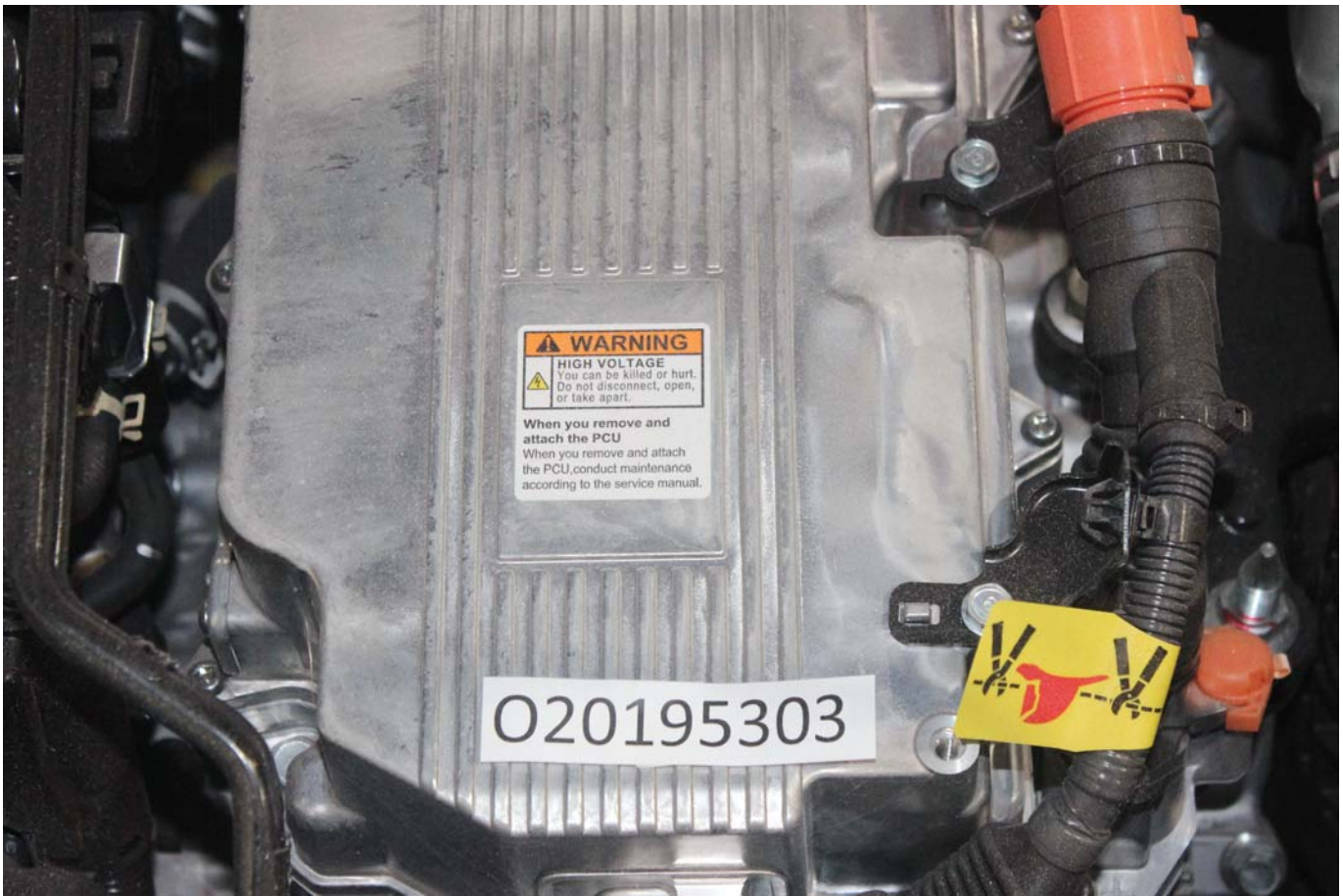
Photo No. 003 - First Responder Warning Label
