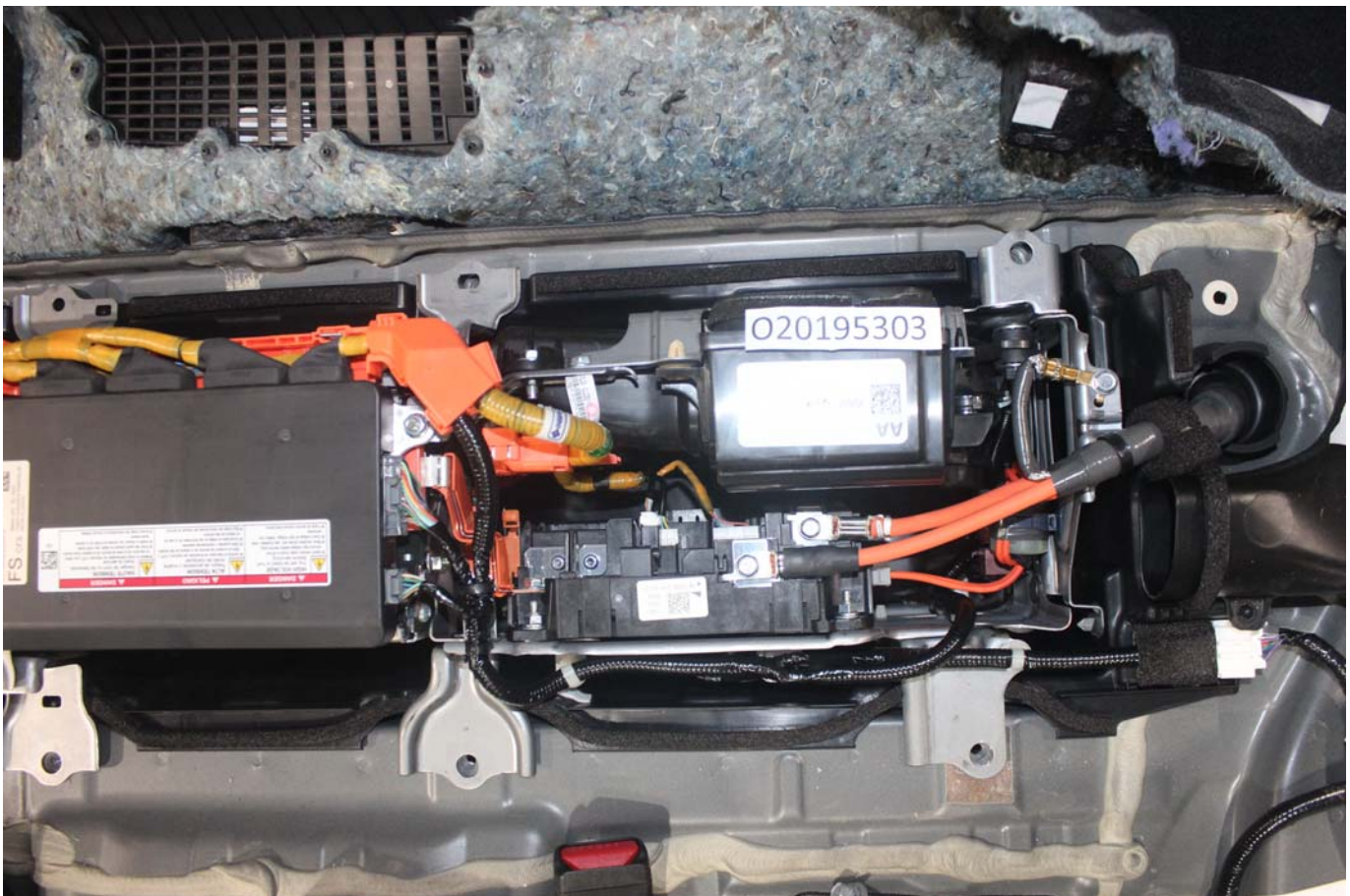
Photo No. 017 - Pre-Impact View of High Voltage Interconnect(s)
