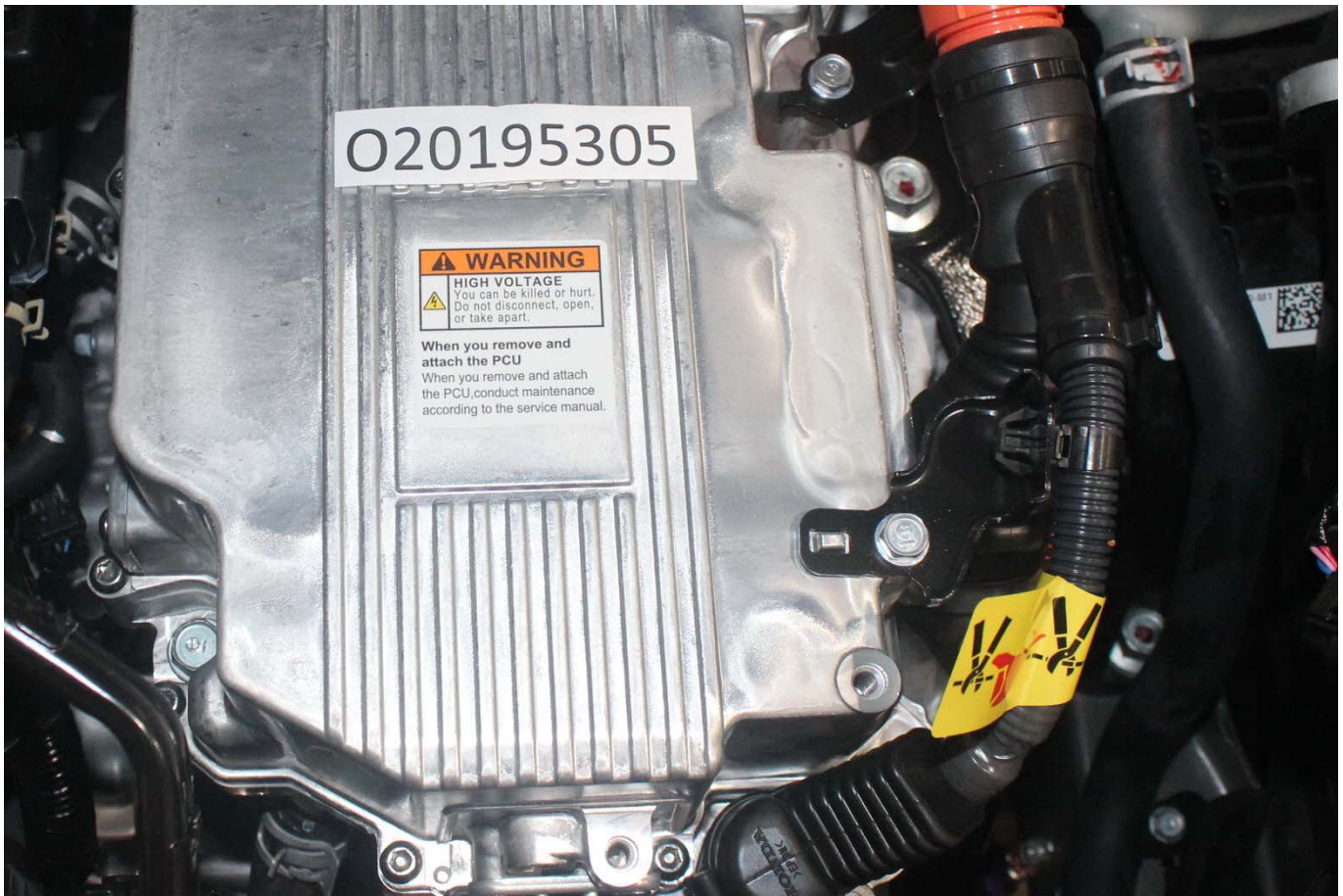
Photo No. 003 - First Responder Warning Label
