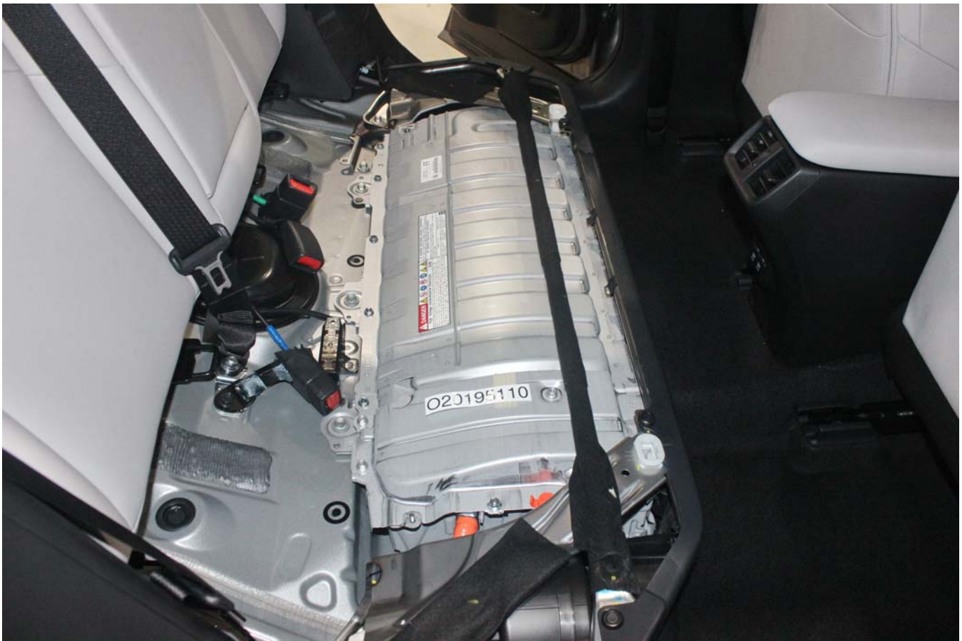
Photo No. 008 - Pre-Impact View of Propulsion Battery
