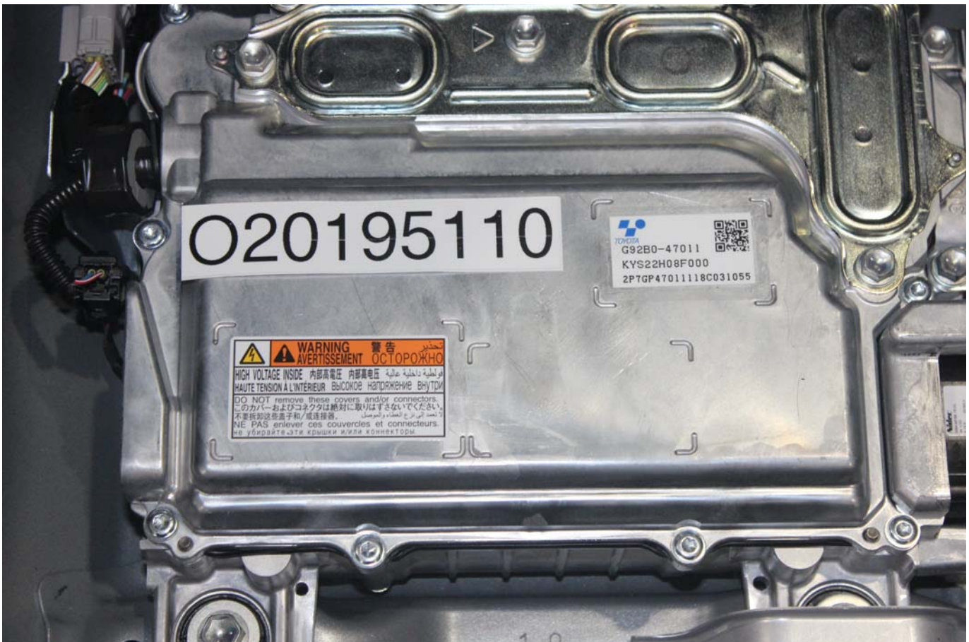
Photo No. 002 - Power Inverter Warning Label
