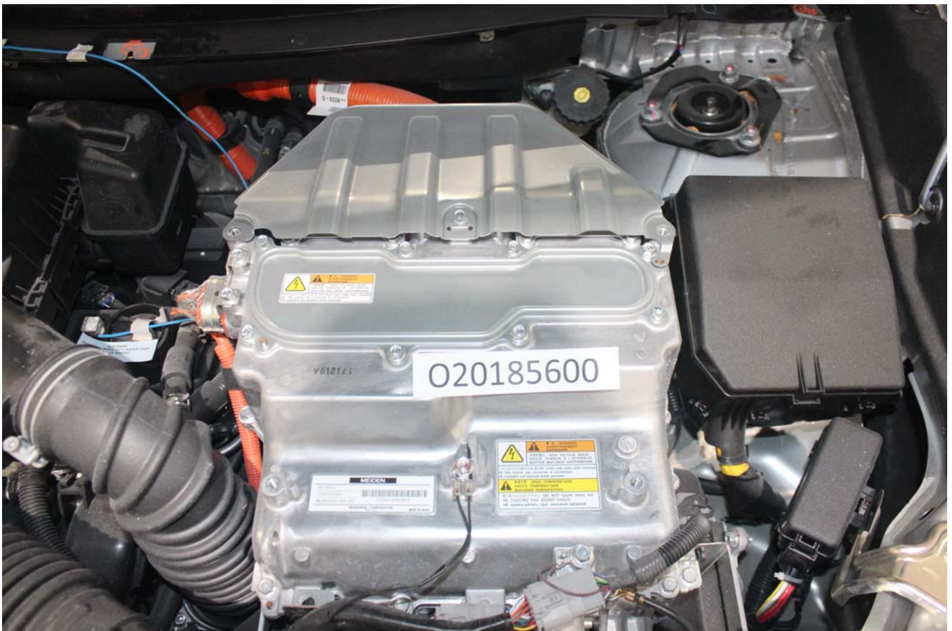
Photo No. 002 - Power Inverter Warning Label
