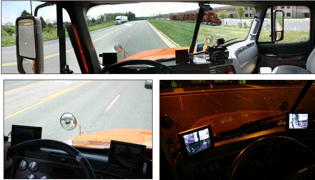
Figure 75. Commercial C/VIS's Monitor Installation
