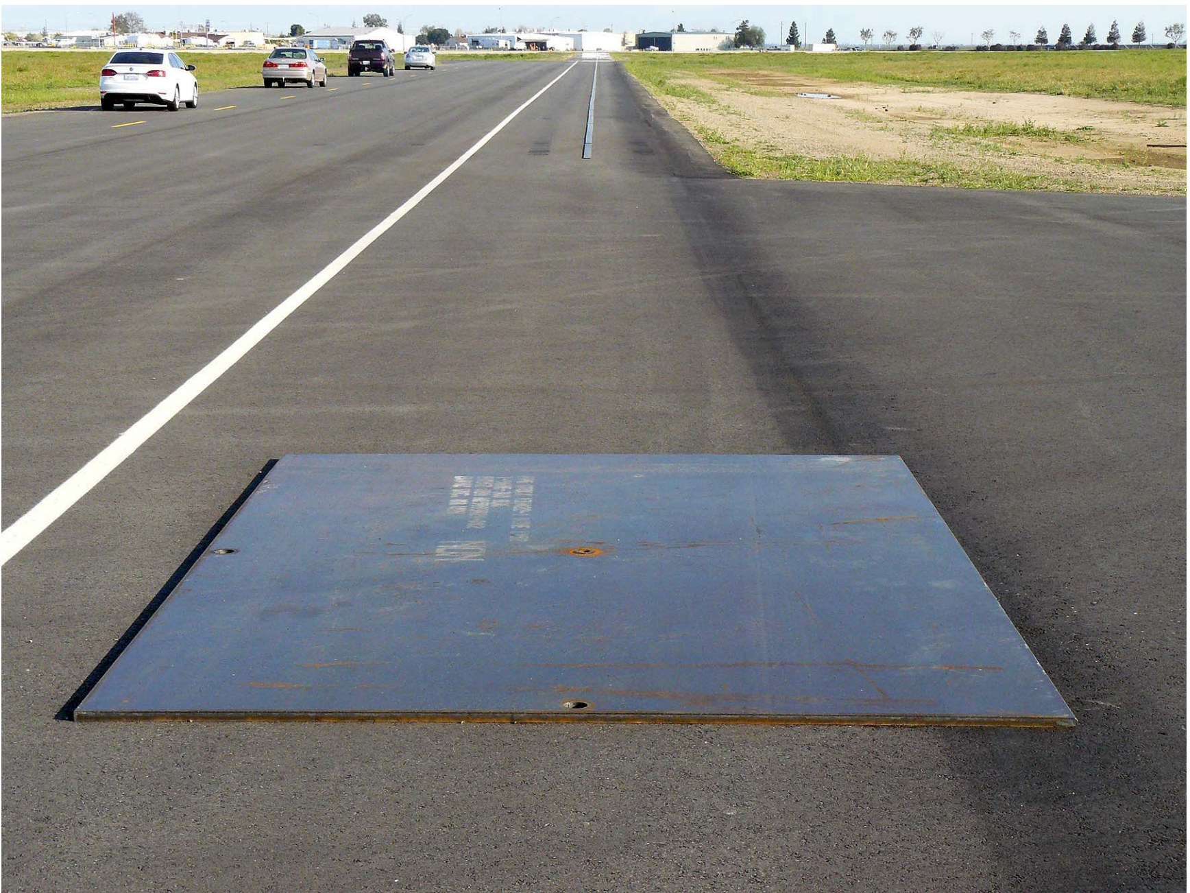
Figure A9. Steel Trench Plate
