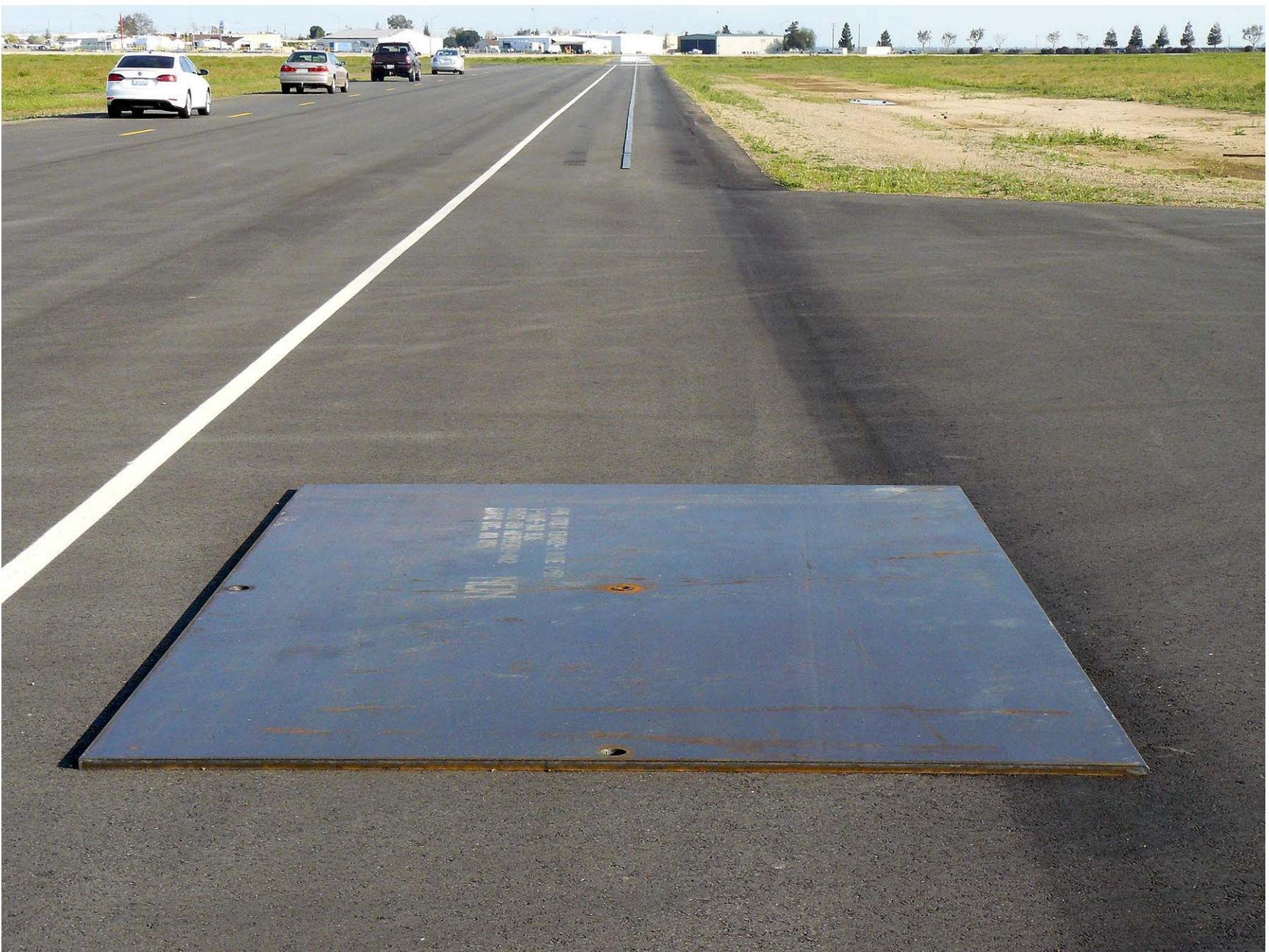
Figure A9. Steel Trench Plate
