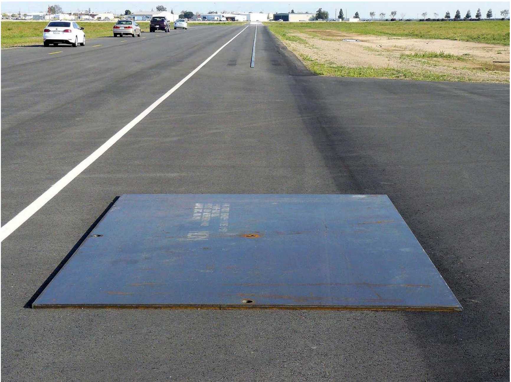
Figure A9. Steel Trench Plate
