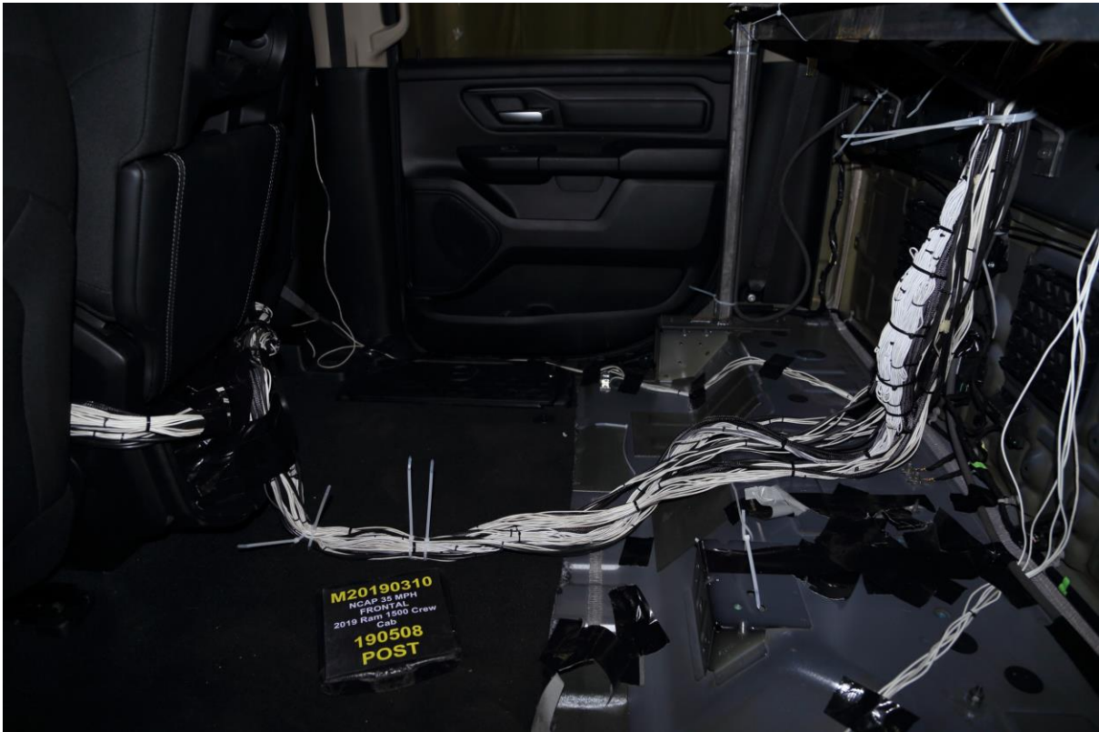
029 Post-Test Dummy Cable Routing
