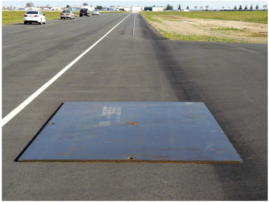
Figure A9. Steel Trench Plate
