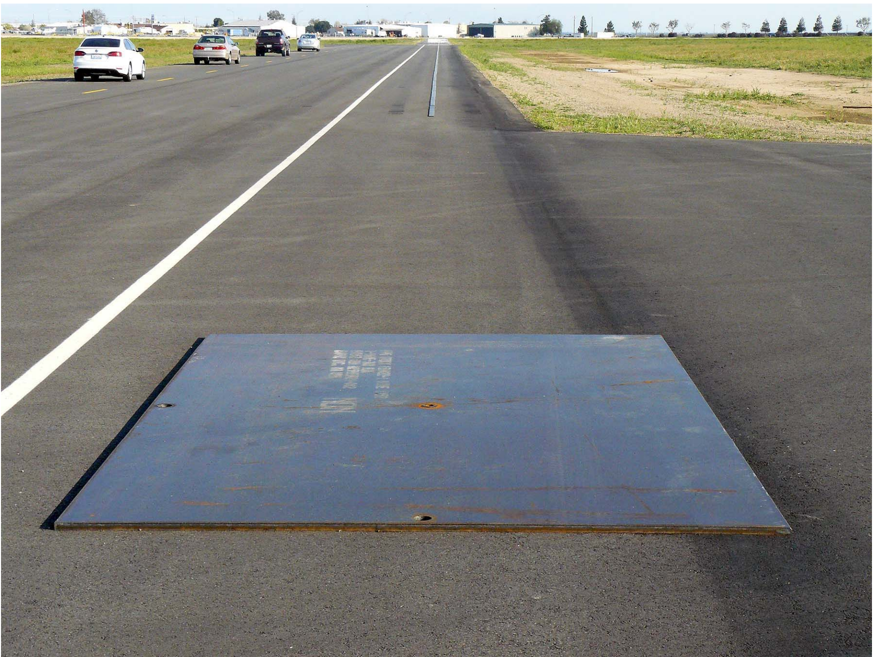
Figure A9. Steel Trench Plate
